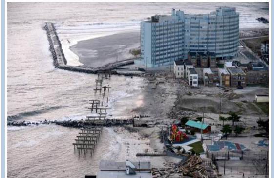
A boardwalk and waterfront property were heavily damaged following Hurricane Sandy in Atlantic City, N.J. One year later, some businesses are still unprepared for disaster, while others have been spurred to make changes. © MICHAEL REYNOLDS
