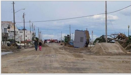
Hurricane Sandy Damage, North End of Brigantine, New Jersey
