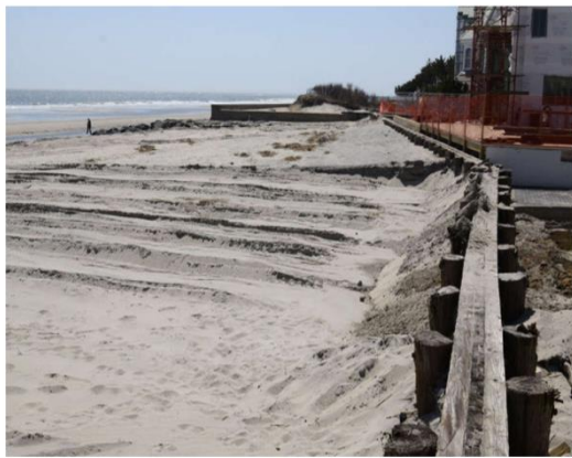
A section of beach at 24th Street in Longport, where there are no dunes. The borough has already suffered $10 million in public property damage. (TOM GRALISH / Staff Photographer)
