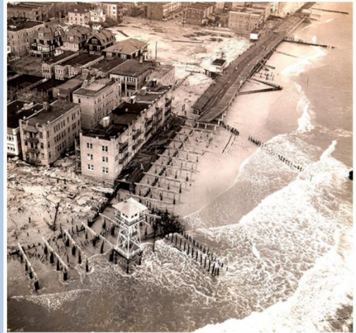
Storms have caused significant damage to Atlantic City's iconic boardwalk throughout its existence. Shown here is South Inlet during the Great Atlantic Hurricane of 1944. (Archive of the Beach Erosion Board stored at the Coastal and Hydraulics Laboratory, Engineer and Research Development Center, Vicksburg, Mississippi, USA)
