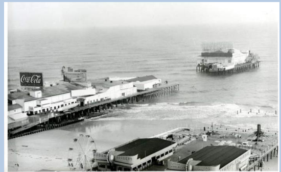
The March 1962 Nor'easter destroyed a section of the Steel Pier in Atlantic City (Photo courtesy of the archives of the Daily Journal).
