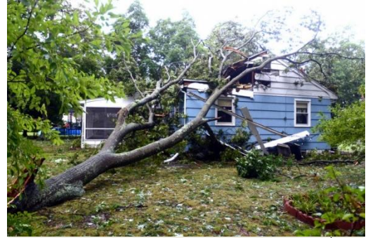
A large section of a tree fell on this home on 2 nd Avenue in Northfield, causing severe damage during Hurricane Irene. (Anthony Smedile)
