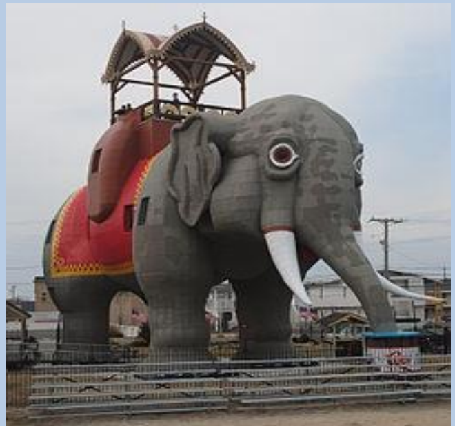
Lucy the Margate Elephant, a National Historic Landmark built in 1881 by James V. Lafferty, has been struck twice by lightning in recent years, once in 2007 and again in 2011 (photo courtesy Wikipedia)
