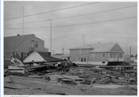
Damage in Longport from the March 1962 Nor'easter. Photo courtesy of the Stewart Farrell Collection.
